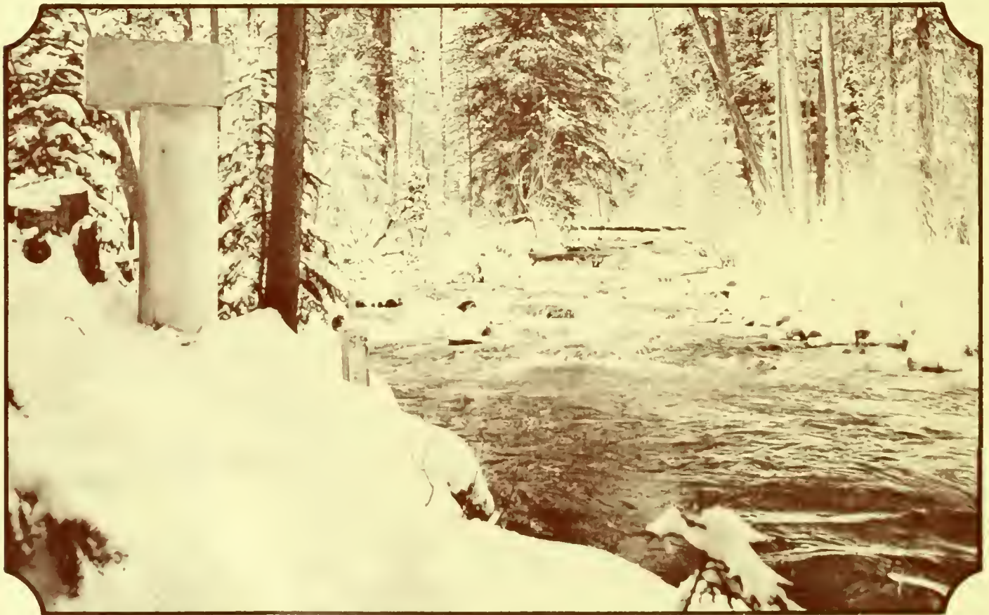
STREAM-GAGING STATION ON NORTH MEADOW CREEK, NORTHWEST OF ENNIS
